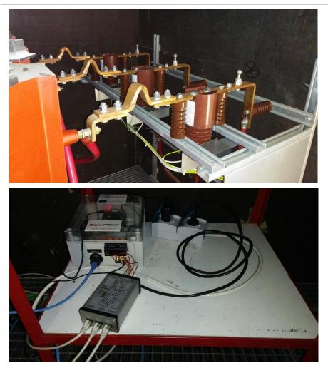
Smart Terminator ALTEA Installed in an RWTH Substation (no need of service interruption)
